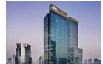
JING AN KERRY CENTRE Shanghai
